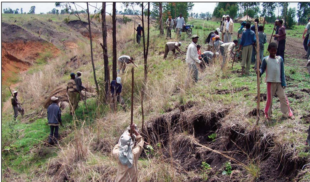
Gully Restoration: Over-grazing is a major problem throughout the Horn of Africa. Resulting erosion has formed deep gullies across the land. Growers are now using the “cut-and-carry” system to maintain their herds while the gullies, protected by trees, vetiver and forage grasses, are coming back to life, sustainably producing high quality forage. The land is coming back to life and the livestock are more productive.
