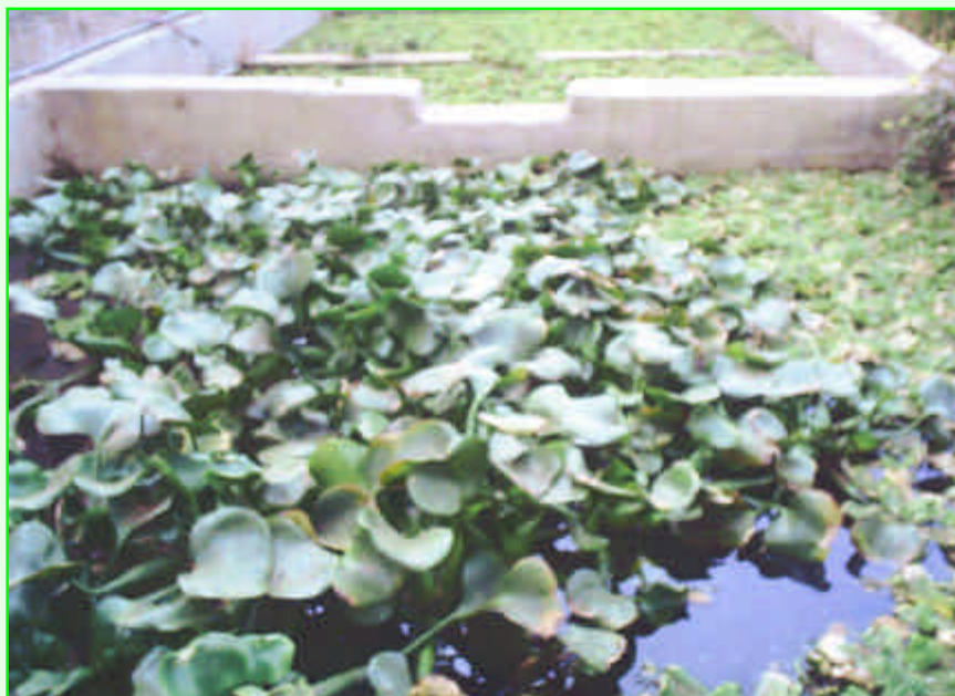
Though slightly out of focus, here is a close-up shot of the sequence of Brandy's retention pools in the lot behind her apartment building. In the first one you can see the large leaves of the water hyacinths.
